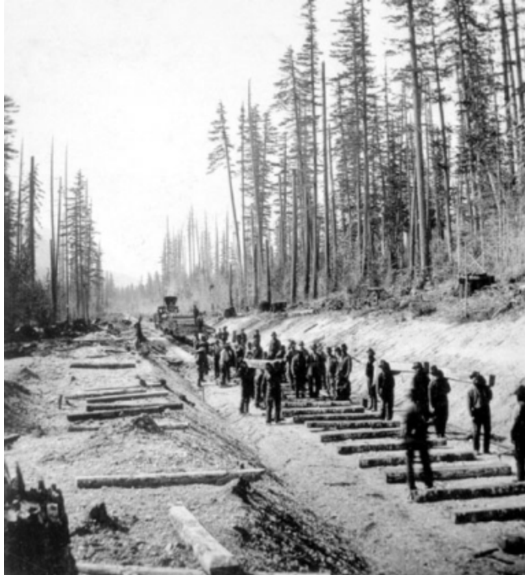
Chinese Railway Labourers building the CP line through the Rockies
