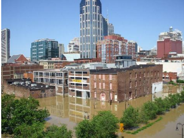
Figure 2: Downtown Nashville buildings under water
